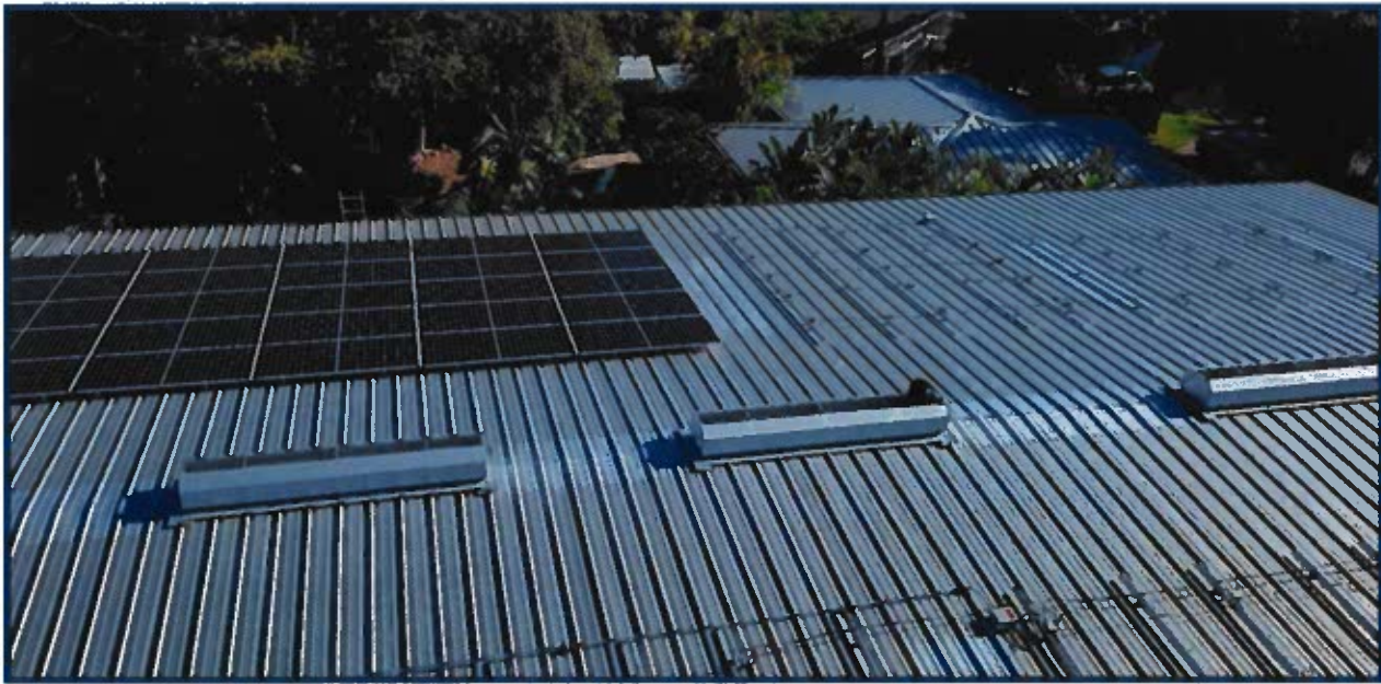
City of Indian Rocks Beach Public Services garage roof
